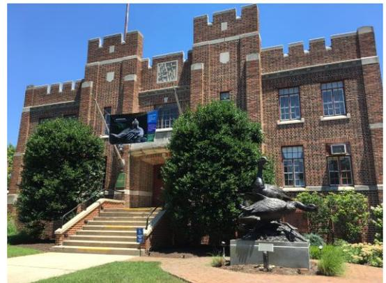
Working closely within MHT guidelines, Waterfowl Chesapeake will hire a contractor specializing in historic restoration. The steel-frame windows will be removed and taken off-site where they will be carefully dismantled, cleaned, repainted and re-glazed before being reinstalled. Work is expected to start in fall of this year.
